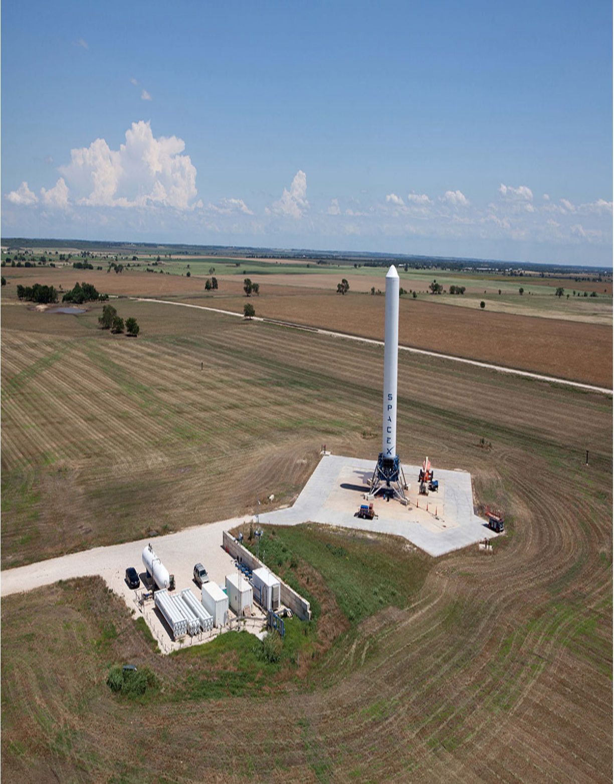
The SpaceX facility in McGregor, Texas.
